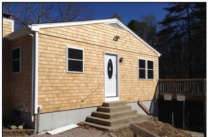
*The WPWA office building's exterior during the winter facelift (top photo by David Smith) and nearing its completion in the beginning of April (bottom). New windows, doors, cedar shingle siding, and roofing completed the exterior work.*
