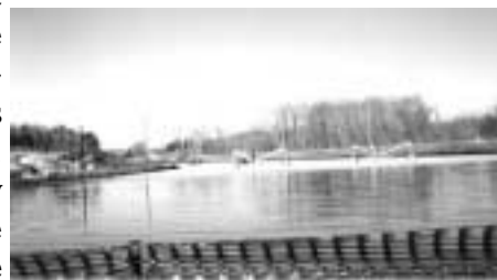
Wastewater treatment lagoon at Kenyon Industries.
