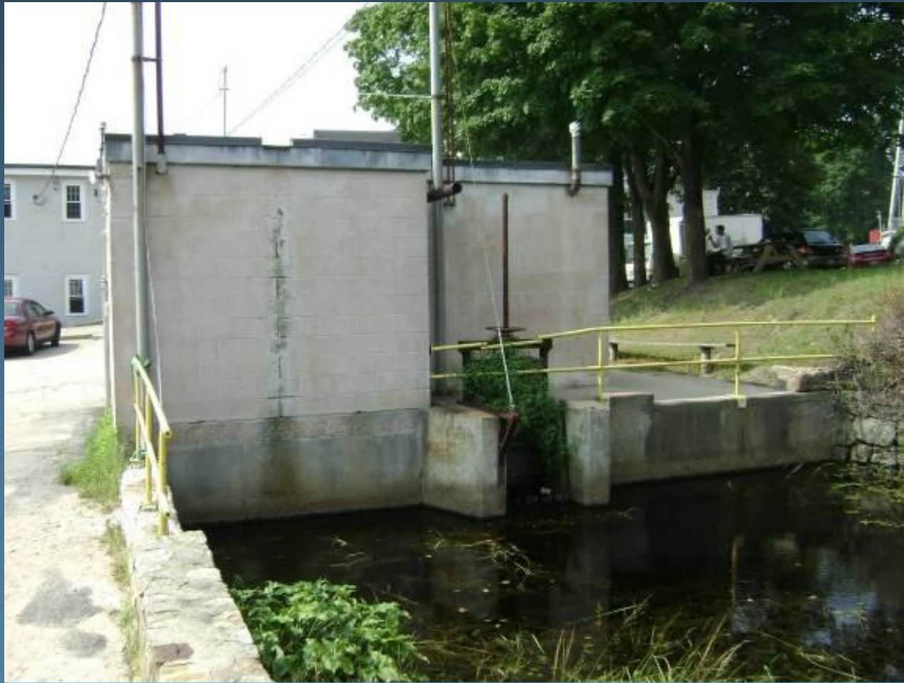
Mill Fire Suppression System Intake - August 2009
