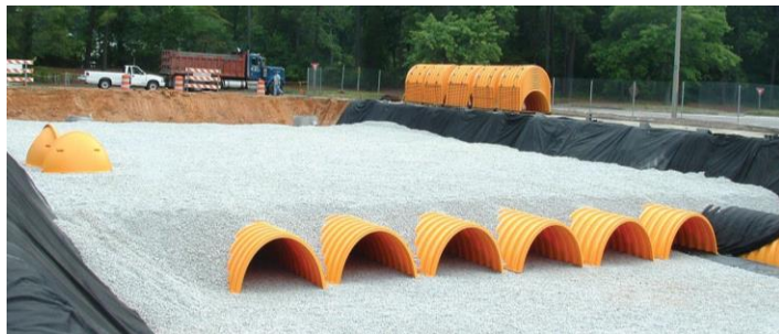
Image 2: Typical installation of underground infiltration system below an existing parking lot. (Image source: stormtech.com)
