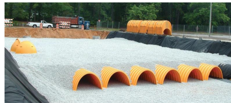
Image 4: Typical installation of underground infiltration system below an existing parking lot. (Image source: stormtech.com)
