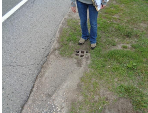
Image 1: View of catch basin located along roadside where proposed BMP would be located. Note the sediment loading and need for maintenance.
