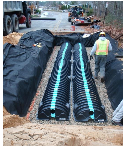
Image 1: Typical installation of underground infiltration chambers beneath a roadway. (Image source: http://capecodwatershed.blogspot.com/ )
