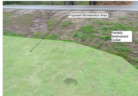
Image 1: View of proposed bioretention area and location of outfall partially filled-in with sediment located in a traffic island adjacent to Carolina Back Road, Charlestown, RI.
