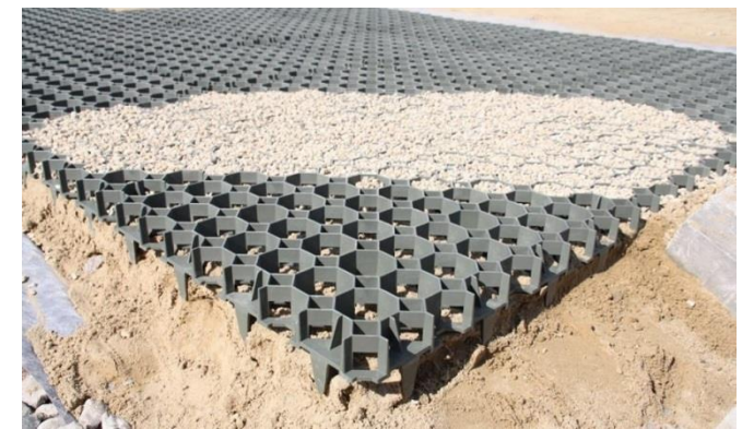
Image 5: View of a typical porous paver profile. (Image source: http://therubbercompany.com )
