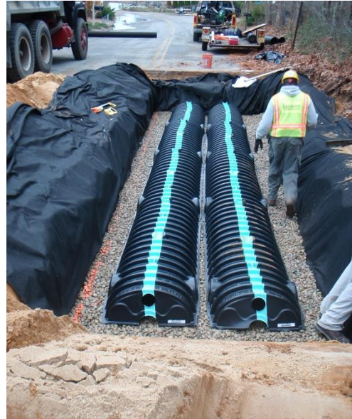
Image 2: View of typical linear infiltration chamber installation beneath a road, Mashpee, MA. (Image source: http://capecodwatershed.blogspot.com/ )
