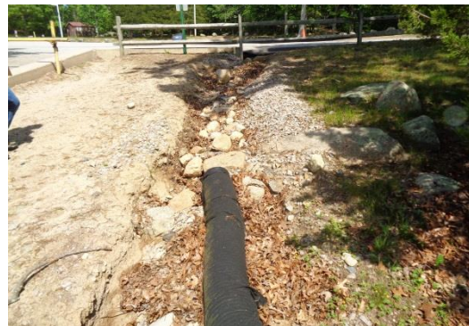
Image 2: View of current outlet exiting parking area. Note erosion along embankment.
