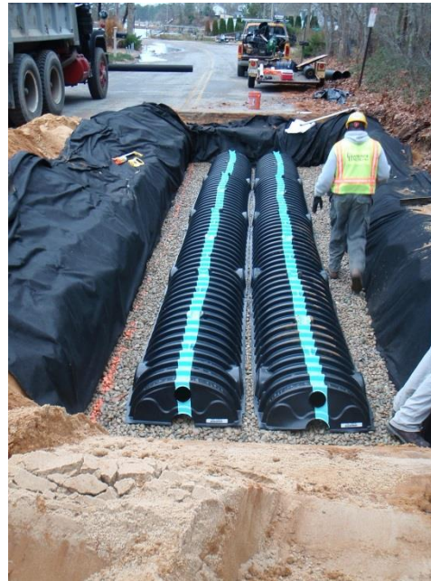
Figure 1: View of typical linear infiltration chamber installation beneath a road, Mashpee, MA. (Image source: http://capecodwatershed.blogspot.com/ )
