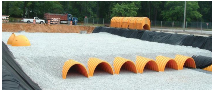
Image 1: Typical installation of underground infiltration system below an existing parking lot. (Image source: stormtech.com)
