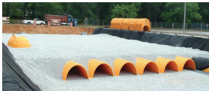
Image 4: Typical installation of underground infiltration system below an existing parking lot. (Image source: stormtech.com)
