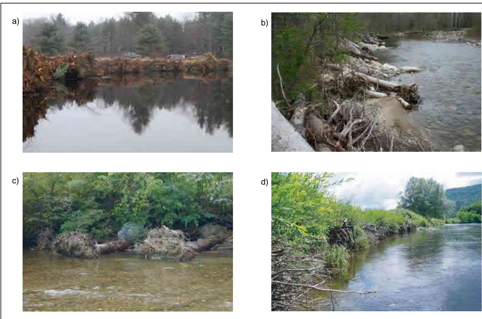
Figure 10. Examples of bioengineering techniques for bank stabilization include use of a) marginal log jams (Souhegan River in Merrimack, NH), b) boulder and log deflectors (Sunday River in Newry, ME), c) root wad revetments (Batten Kill in Arlington, VT), and d) willow stakes above root wad revetment (Connecticut River in Colebrook, NH).
