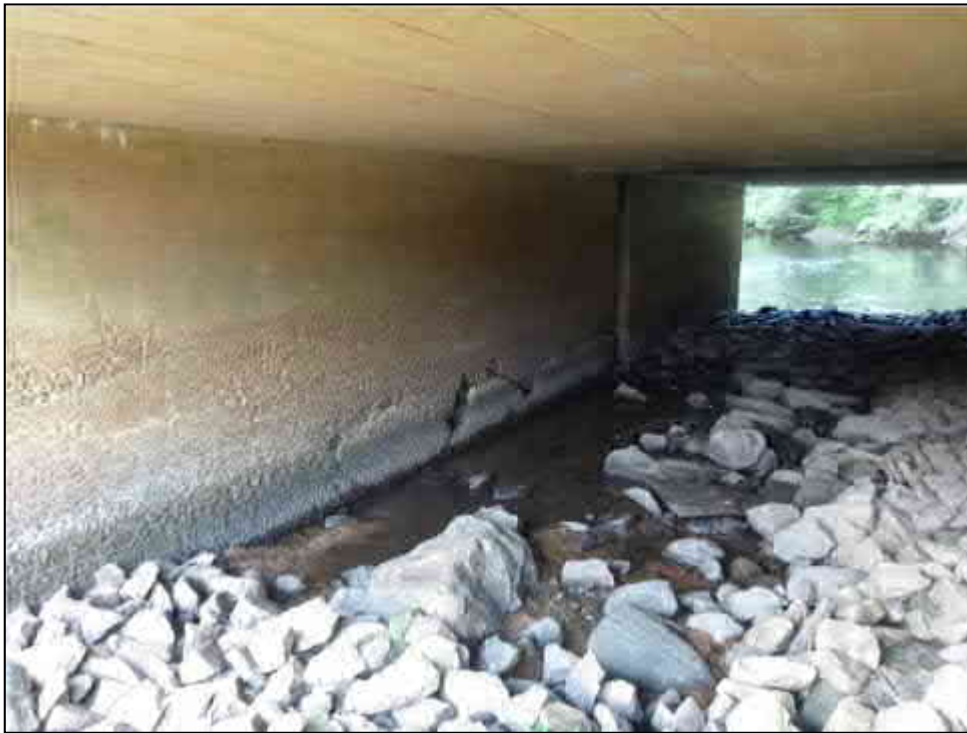
Figure 13. Old Shannock Road Bridge in PAR-23 showing a) upstream overview and b) close up of scour damage and subsequent riprap protection.
