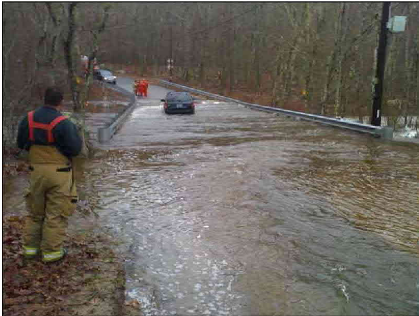
Figure 12. Hillsdale Road overtopped due to backwatering behind undersized culvert during 2010 flood on Beaver River in Richmond, RI.
