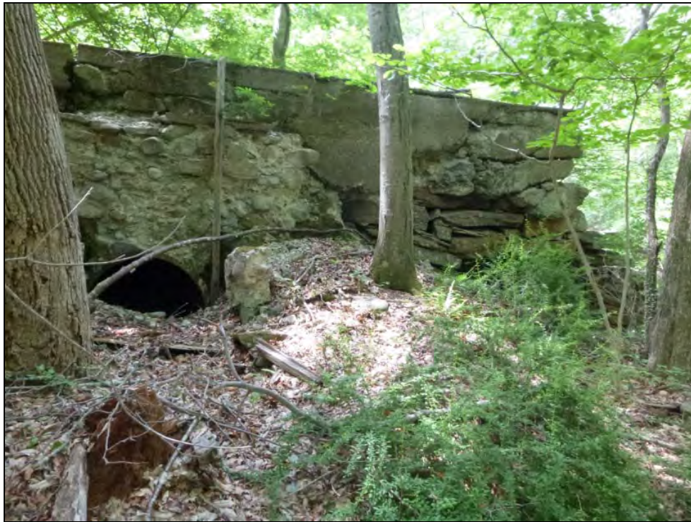
Figure 19. Old dam structure on left bank of GAS-8 showing a) downstream view of structure and b) close up of mill race intake.
