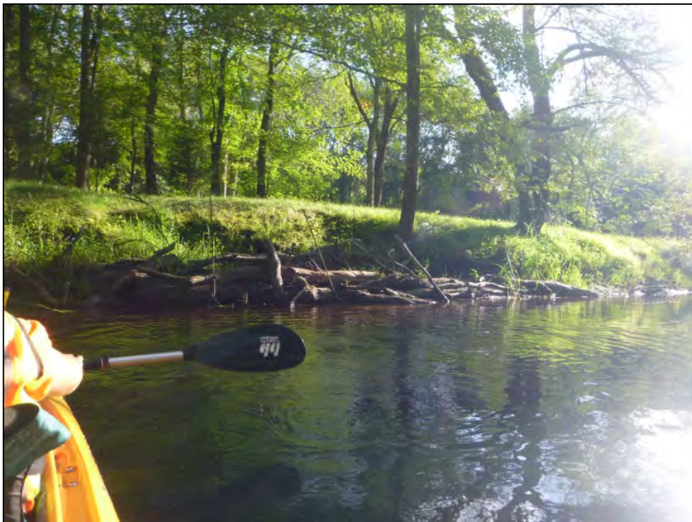
Figure 11. Previous bank restoration efforts in PAR-23 include a) boulder supported marginal log jam structure and b) toe wood revetment. Views looking downstream.
