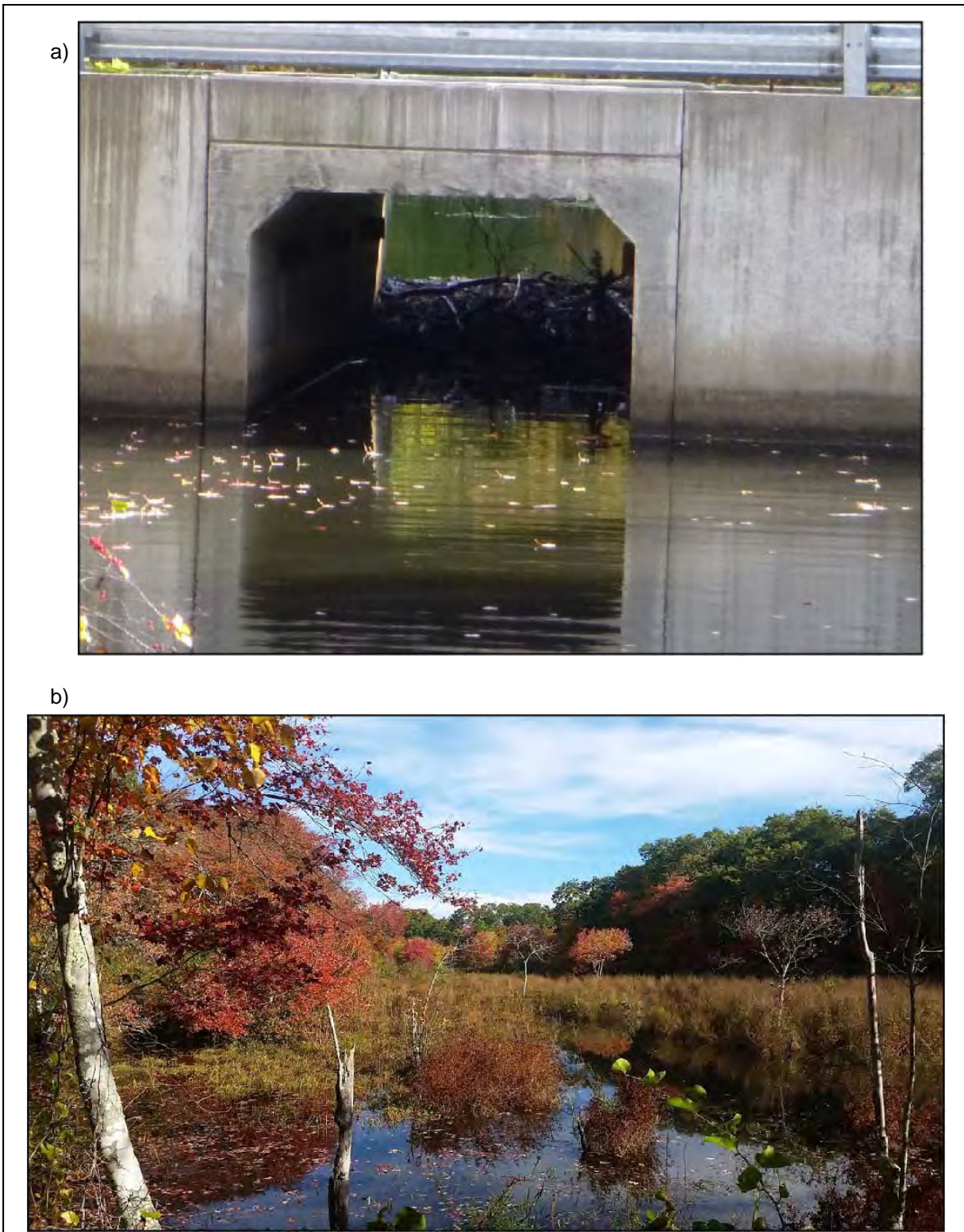
Figure 7. a) Upstream view of the beaver dam in the undersized culvert at Wolf Rock Road in Exeter, RI (CHIP-8) and b) upstream view from road of beaver meadow wetland.
