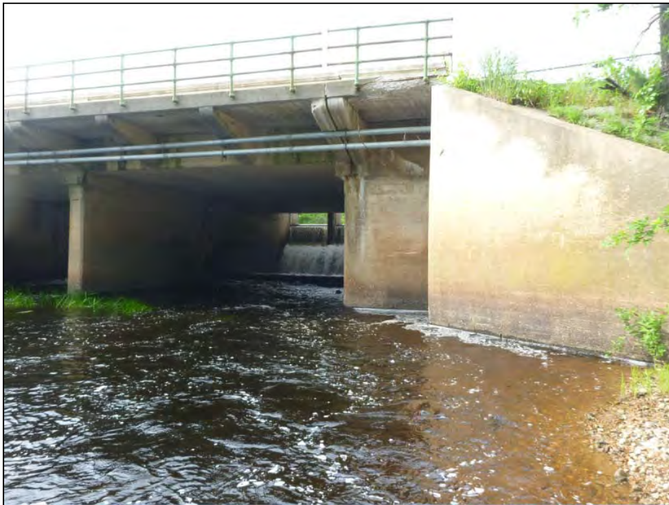
Figure 18. Route 91 Bridge and Alton Dam in WOR-1 showing a) right bank view of pier scour and b) dam underneath bridge.
