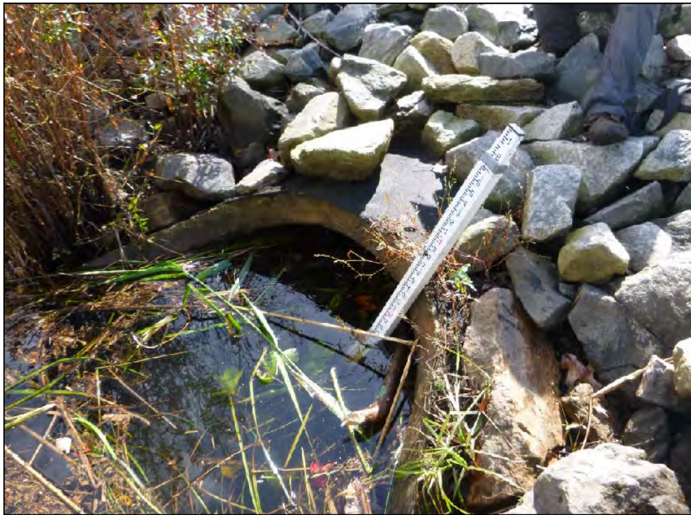
Figure 26. Undersized culvert at Yawgoo Valley Road in CHIP-8 showing a) upstream view of entire crossing and b) close up of beaver dam clogging culvert inlet.
