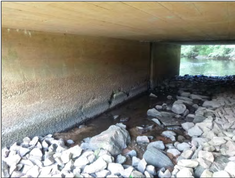
Figure 10. a) Downstream view of Old Shannock Road Bridge in PAR-23 and b) closeup of riprap placed on bed and scour of bridge pier in right bank cell.
