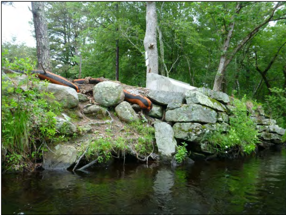
Figure 16. a): Downstream view of old abutments constricting channel in WOR-16 and b) right bank view of bank erosion due to abutments.
