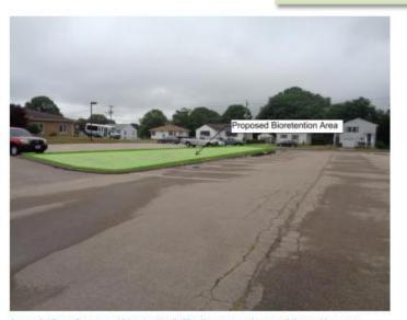
Image 3: View of proposed bioretention/infiltration area and some of the parking area that would drain to it.
