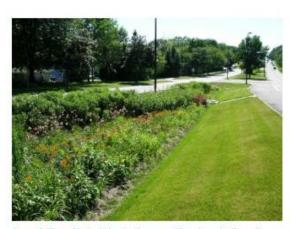
Image 3: View of typical bioretention area with mature plantings. (Image source: http://www.installitdirect.com/wp-content/uploads/2015/01/how-to-build-a-rain-garden.jpg)
