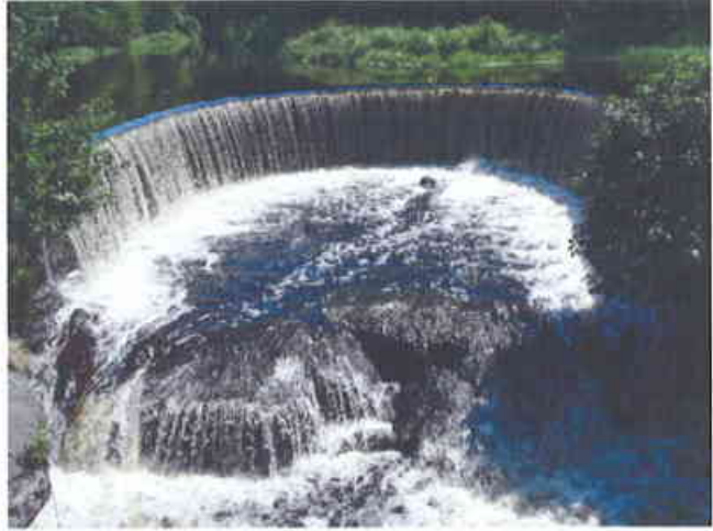
View of Upper Shannock Horseshoe Falls Dam looking upstream
