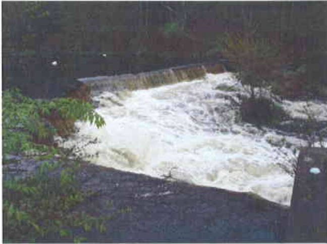
View of Lower Shannock Falls Dam from the right bank
