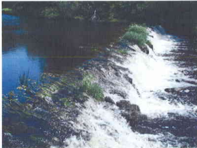
View of Kenyon Mill Dam from the right bank
