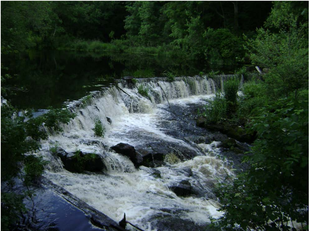
Lower Shannock Falls Dam
