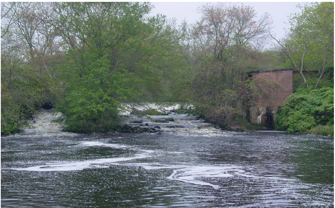
Lower Shannock Falls Dam
