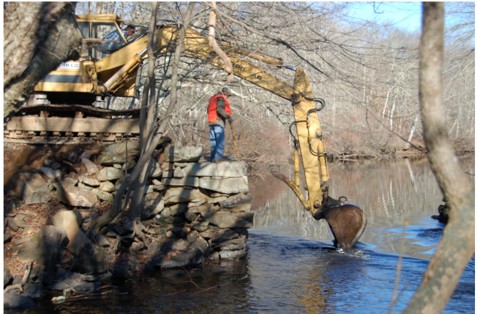
Contractor restoring the Hopkinton abutment of the bridge prior to installation of the new pedestrian bridge. (Photo courtesy of H. Buford.)
