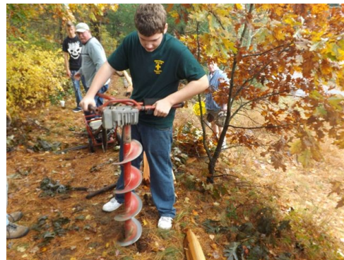
Drilling holes for the 300 yard long fence.
