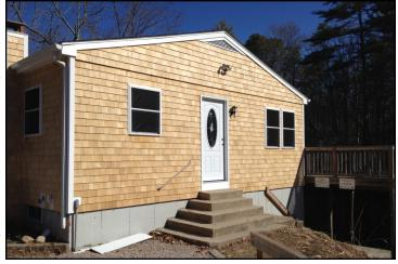
The WPWA office building's exterior during the winter facelift (top photo by David Smith) and nearing it's completion in the Phase III and is expected to complete the project in beginning of April (bottom). New windows, doors, cedar shingle siding, and roofing completed the exterior work.
