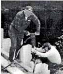
Roy Grinnell and Jim Caswell installing vinyl seawall.
